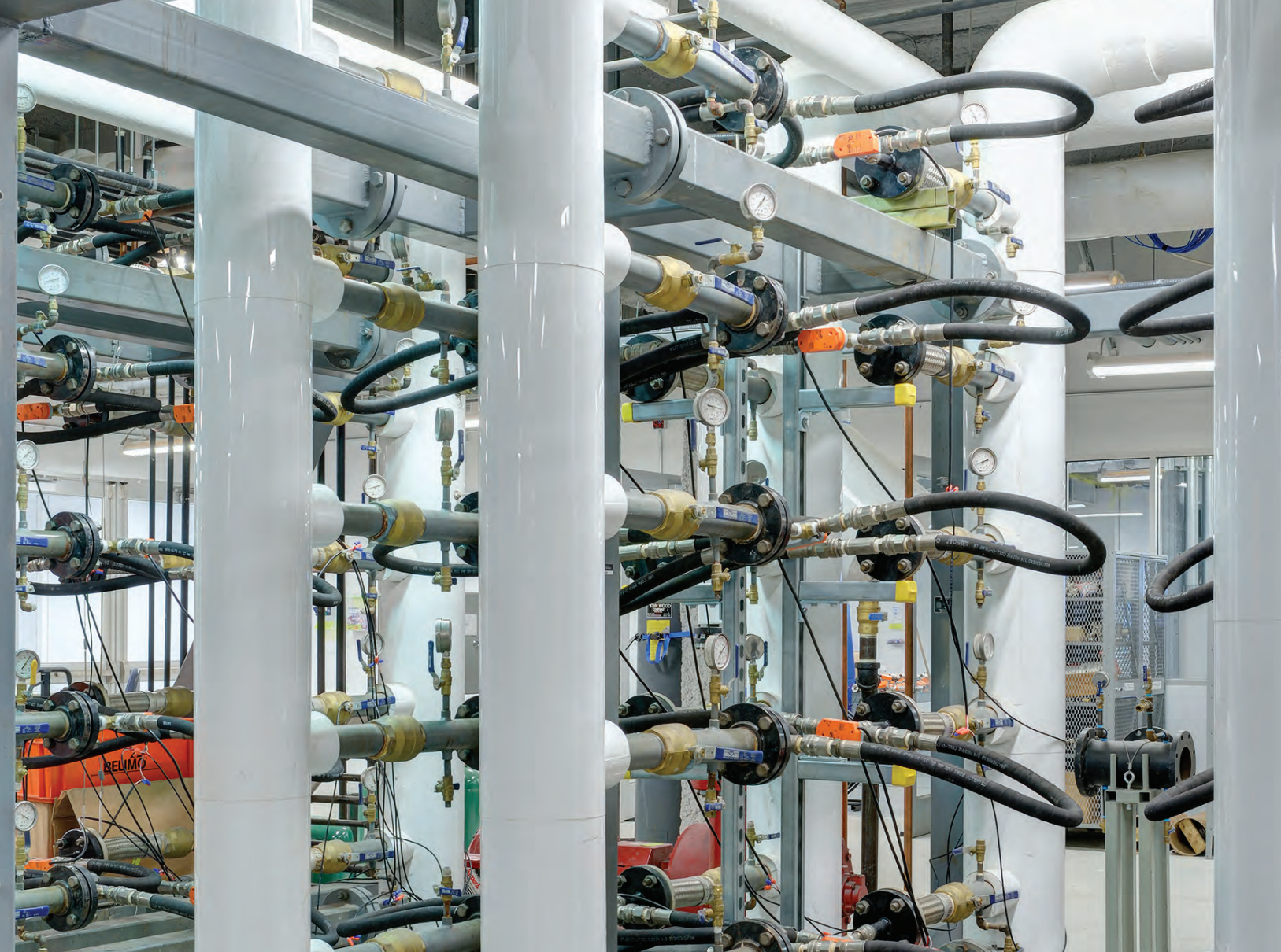
Belimo Americas Headquarters Test Lab, Danbury, CT
